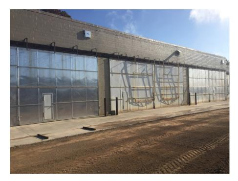
**Figure 5.** These are dehumidification kilns, though it's hard to tell the difference from most other kiln types just by looking at the outside of the building. One difference from large conventional kilns is that the vents are smaller and fewer in number (in this photograph the vents are above the doors at the front of the building). Each of these large kilns holds about 50,000 board feet of lumber.
