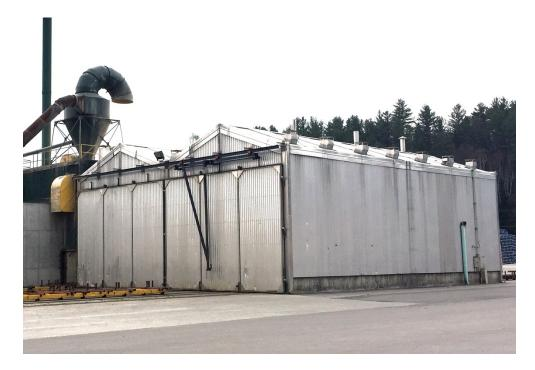
*Figure 1.* Conventional steam-heated dry kilns. There are large doors for loading the lumber in the front of the kiln, and the kiln is constructed from corrosion-resistant materials. Notice the number of vents in the kiln roof. These are used to vent water vapor from the drying lumber.
