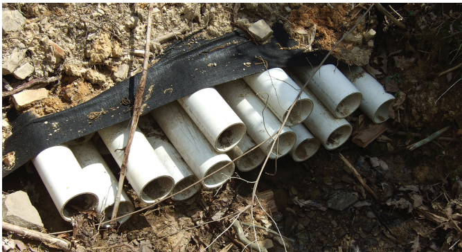
Pipe bundles are one option to use for temporary storm crossings.
